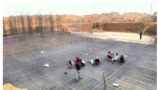
Construction as on 15th May 2016
